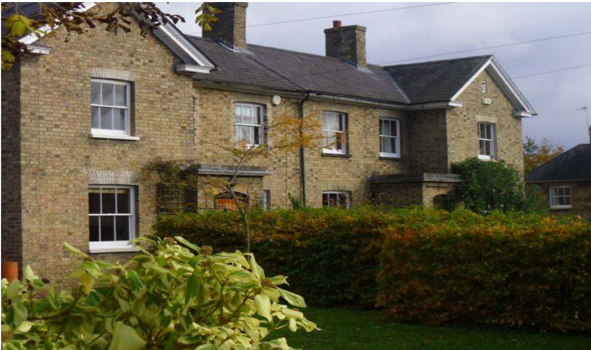
Duke of Bedford Cottages - Oakley
