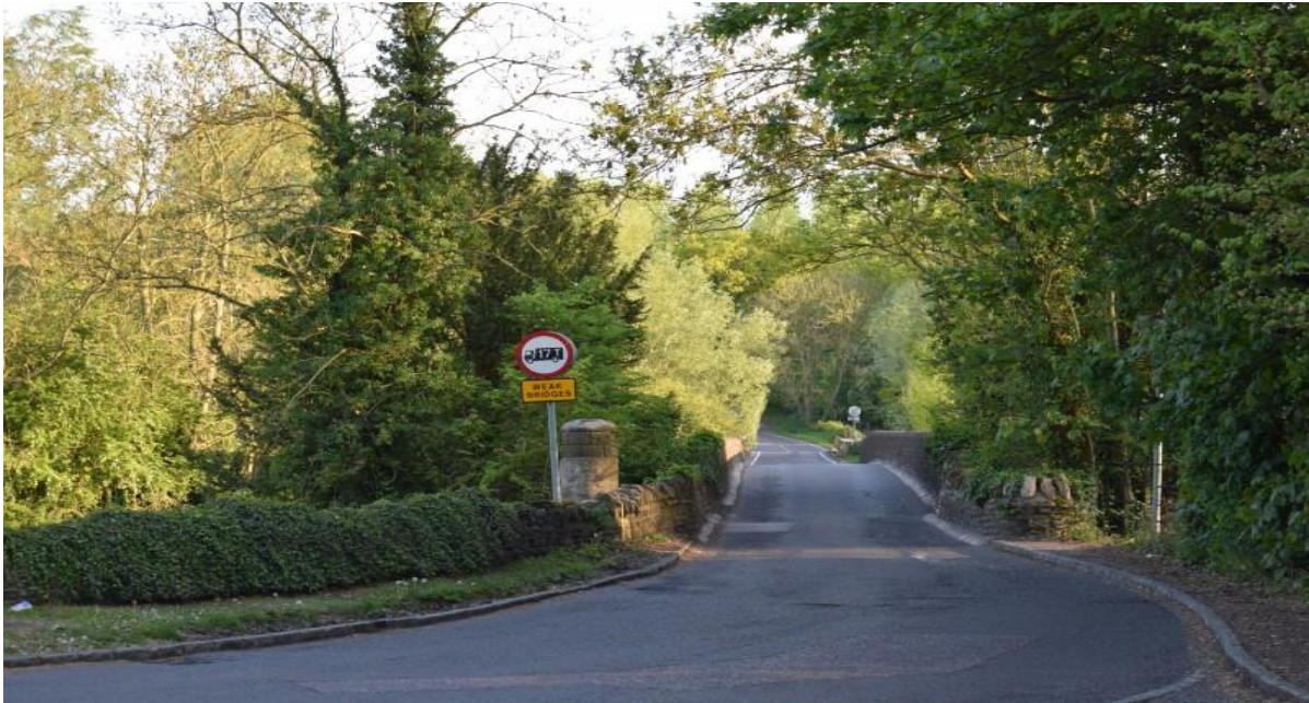
Twin-bridges over the river Great Ouse in Oakley
